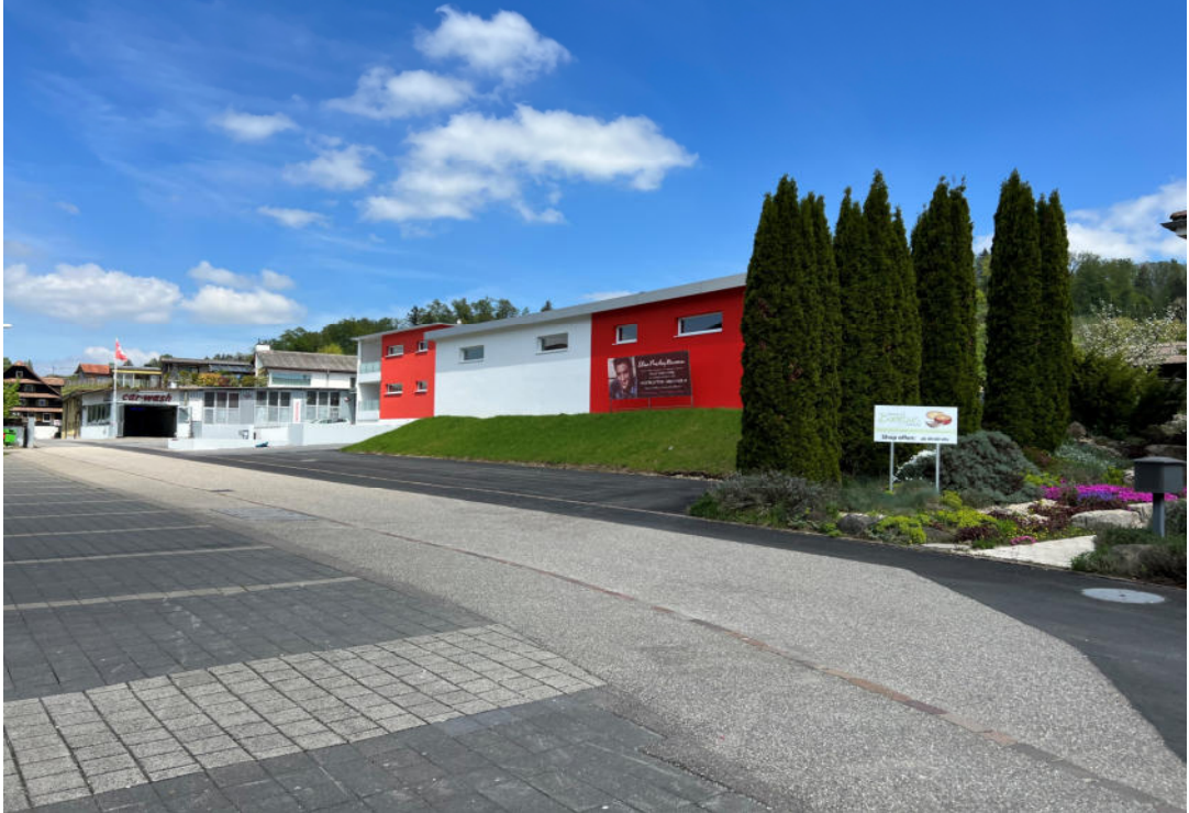
Haus 14 Foto 2 Geschosse 0 G Höhe 5.89 m Fotoname building 14 picture 2 floors height picture name
