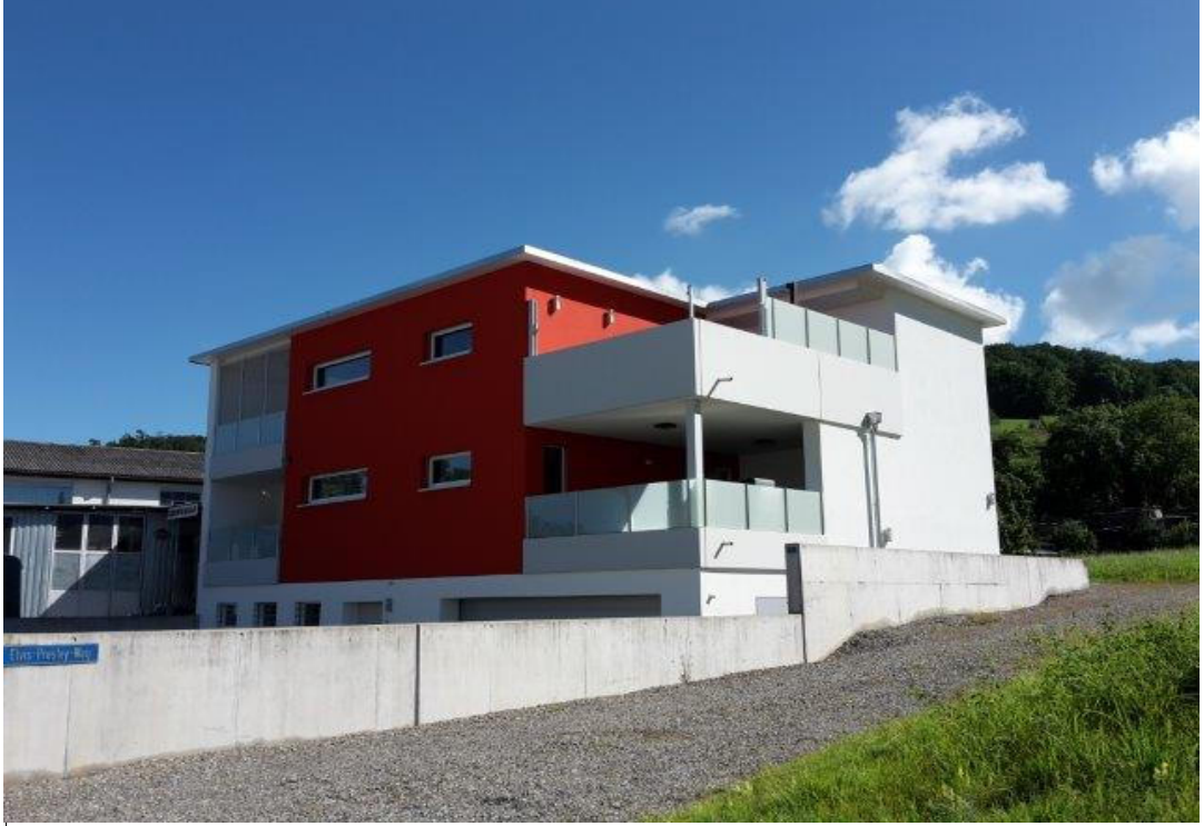
Haus 5 Foto 2 Geschosse 2 G Höhe 7.14 m Fotoname building 5 picture 2 floors height picture name
