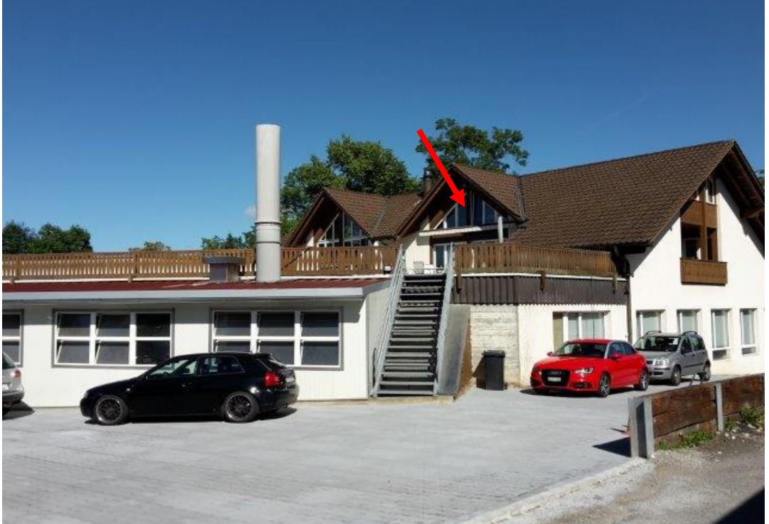
Haus 3 Foto 1 building 3 picture 1 Geschosse floors 2 G Höhe height 5.83 m Fotoname picture name
