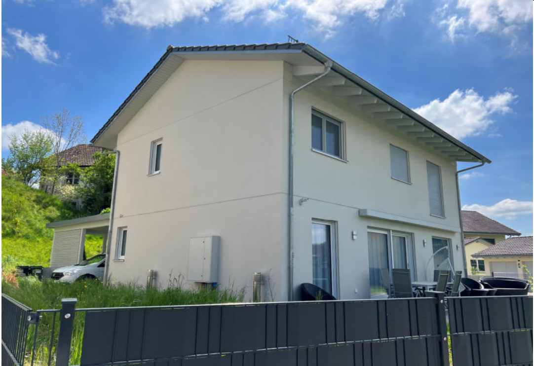
Haus 16 Foto 2 Geschosse 1 G Höhe 4.77 m Fotoname building 16 picture 2 floors height picture name
